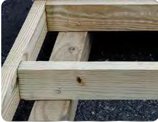
Pressure Treated 2x4 Floor Joists 4x6 Runners
