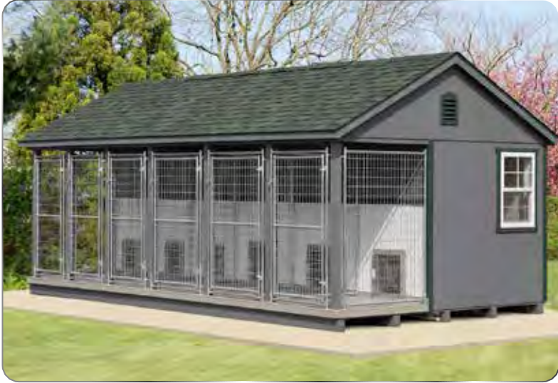
4' High Glassboard on Exterior Run Wall
