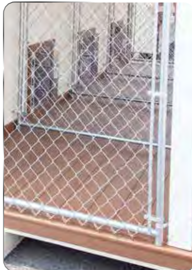
COMPOSITE DECKING ON RUNS
