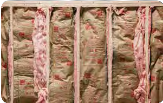
R-13 Batten Insulation In Walls & Ceiling
