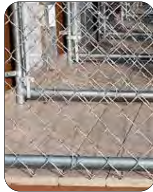
Poly Decking on Runs
